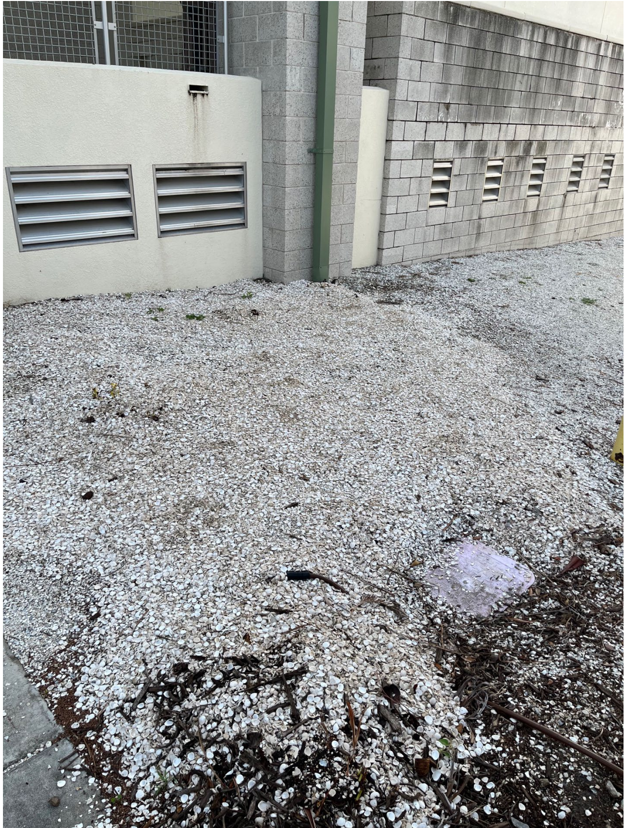
VIEW ABOVE OF CRUSHED SHELL PAVING
